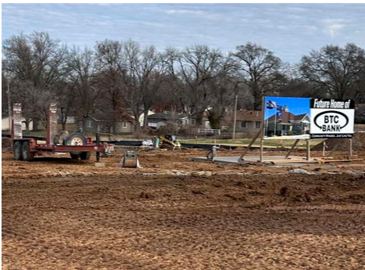
Breaking ground on 16th St. location across from MO State Fairgrounds
